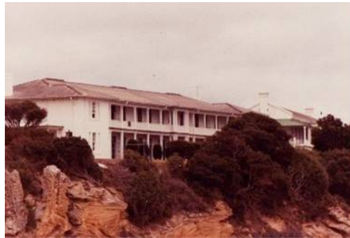
44 Building I – Home of A Company
