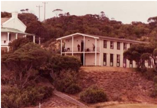
45 Building 6 – Home of B Company
