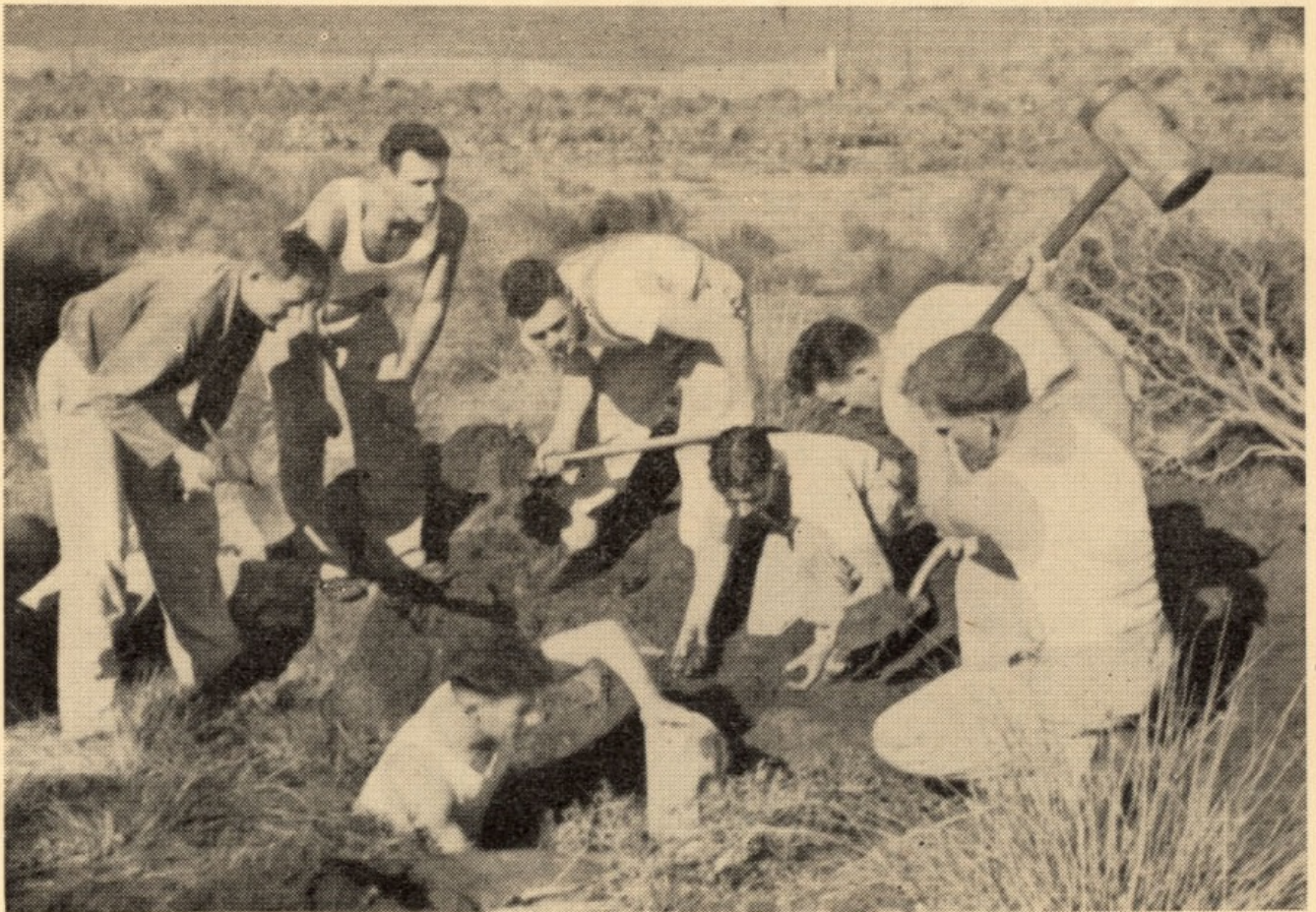
DIGGING WEAPON PITS
